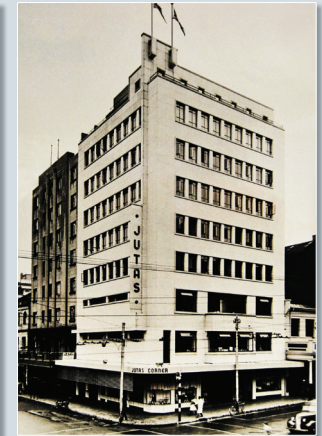
The multi-storey building that still stands on the corner of Loveday and Pritchard in downtown Johannesburg
