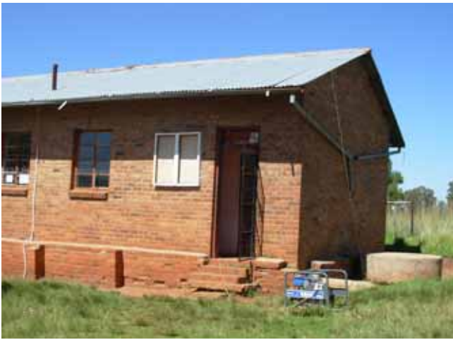
The small generator in front of the administrative block of this rural Eastern Cape School is its only source of power.
