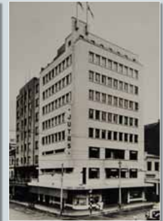
The multi-storey building that still stands on the corner of Loveday and Pritchard in downtown Johannesburg
